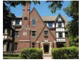
Chapter houses are important assets to upkeep and maintain.
