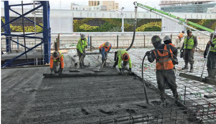
Above & Top Right: Central Concrete Supply Company pouring CarbonCure concrete at UC Hastings, San Francisco.
