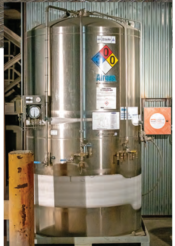
Top: Central Concrete Supply deployed 195 trucks from multiple plant locations to Santa Clara for a large pour.
