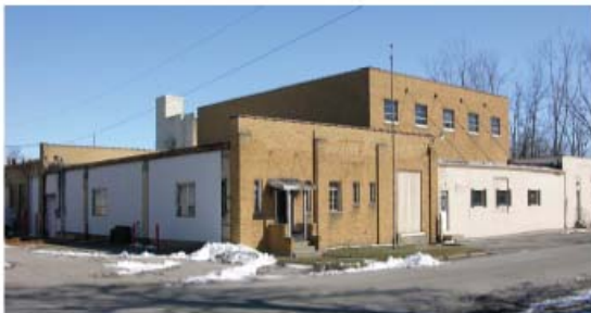
Our new facility located at 1600 E. Washington St. Our dock doors to our regular warehouse are located just to the left in this picture. Photograph taken by Lori Crespo
