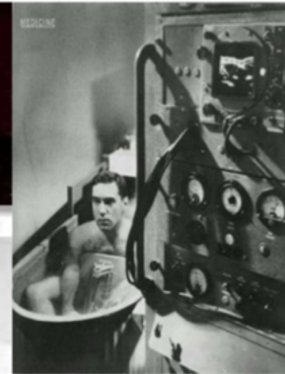
SOUND-WAVE PORTRAIT IN THE FLESH Howrylike device produces pictures of the human body's soft tissues which are invisible to X-rays
