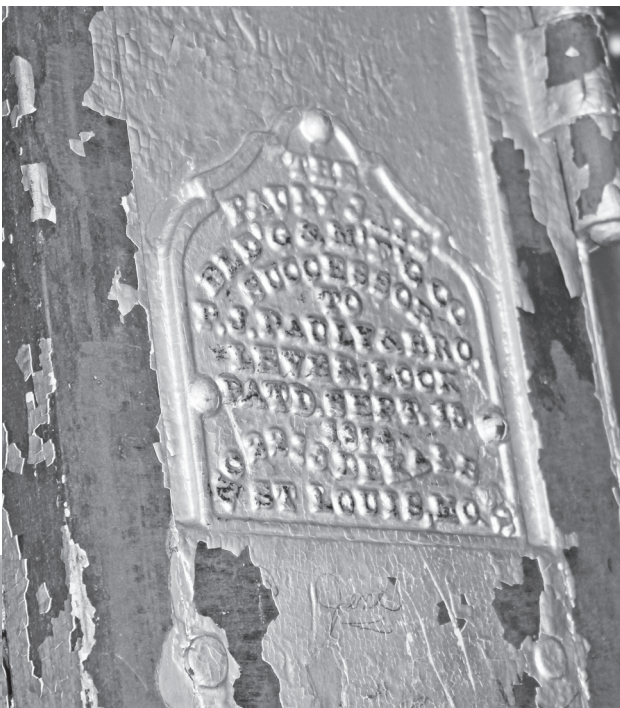
A cast-iron plaque is bolted to the front of the patented locking mechanism outside the jail cells. A lever outside the cell area could lock and unlock the cells without entering the cell area.
