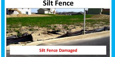
Replace torn, damaged or decomposing silt fence. Remove accumulated sediment that bulges the silt fence or when sediment reaches 1/2 the height of the fence.
