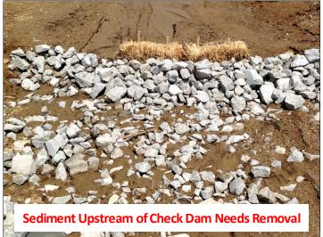
ensure proper flow/operational parameters, То accumulated sediment shall be removed when the sediment reaches ½ the height of the dam.
