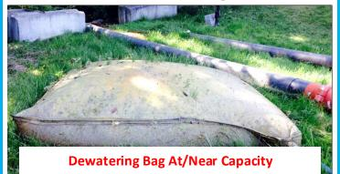
During inspections, check for erosion downstream of the dewatering bag. Check for tears in the dewatering bag; water and sediment capacity.
