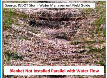
Check for displacement of the blanket and signs of erosion under the blanket. For eroded areas: pull back the blanket; add/tamp soil; re-seed; re-staple blanket.
