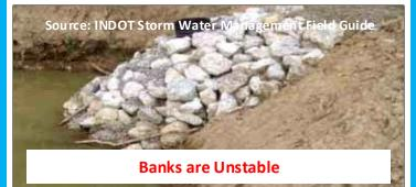
Repair any damage to Principal & Emergency Spillways. If pool area holds water for more than 72 hours, remove/replace filter stone. Remove sediment once design volume is reached (per SWPPP).
