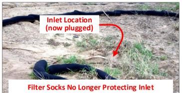
When accumulated sediment reaches ¼ the height of the filter sock, remove the sediment. Repair/replace damaged filter sock. If ponding is excessive, consider alternative BMPs.
