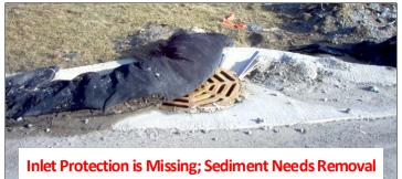
Flushing with water to clean inlet protection is not allowed. After each storm event, remove sediment. If inlet protection measure is repeatedly clogging, consider additional BMPs upstream.
