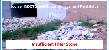
Repair any embankment erosion. If pool area holds water for more than 72 hours, remove/replace filter stone. Remove sediment once sediment trap is ½ full of sediment.
