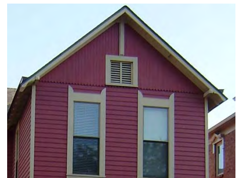
Above, roof line trim board inappropriately boxed in at bottom, Below, done appropriately
